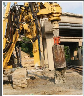
The Pengo cleaning bucket is your go-to option for removing material from the hole to create a clean base. The featured spin bottom ensures whether the bottom is closed or open, preventing spoil spills.
